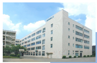
R&D Center in Guangzhou
